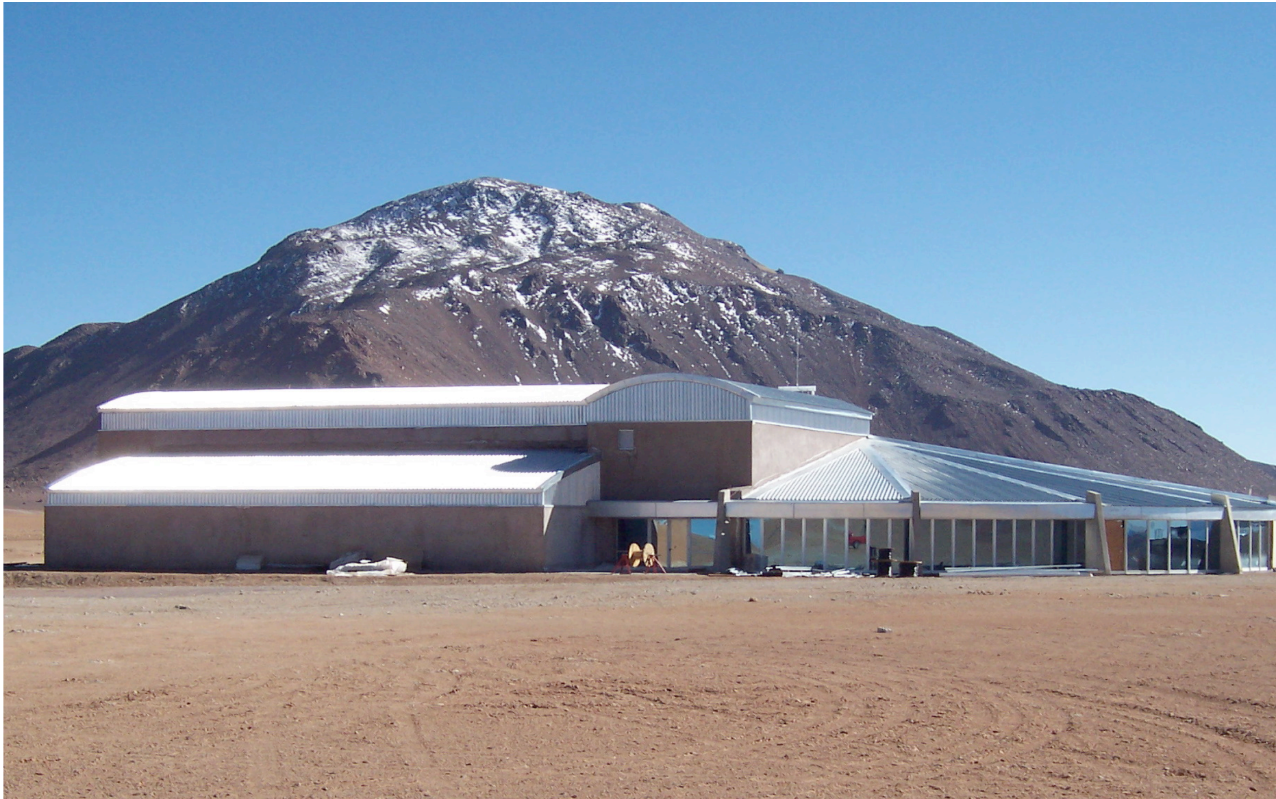
AOS Technical Building – March 2007
